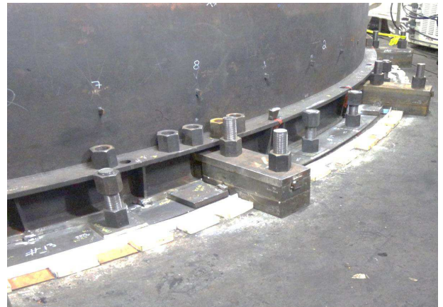
Figure 7 - Assembly before Final Grout
