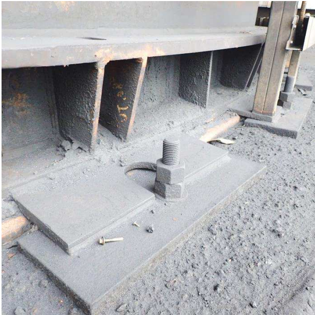
Figure 5 - Early Version of Sliding Restraint
